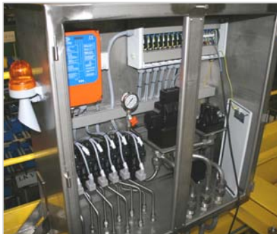
Control box with receiver as electro-hydraulic interface
